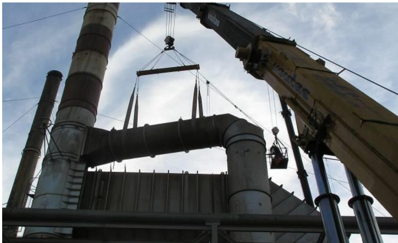
PROJECT: Convection section replacement and maintenance of air preheater 3-H-01 A/B in HEL.PE Refineries in Elefsina
